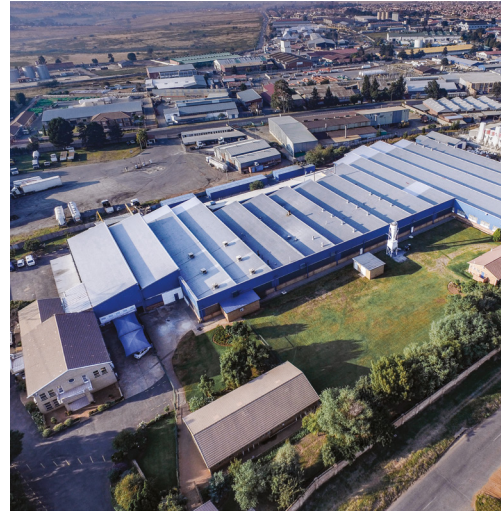
Grinding Techniques headquarters in Chamdor (Krugersdorp)
